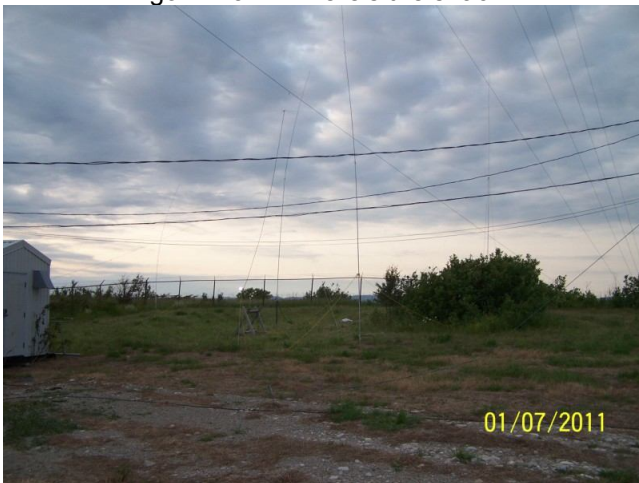
Phased verticals on 40 and 80 antennas
